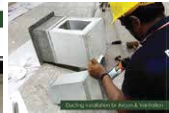
Ducting Installation for Room & Ventilation
